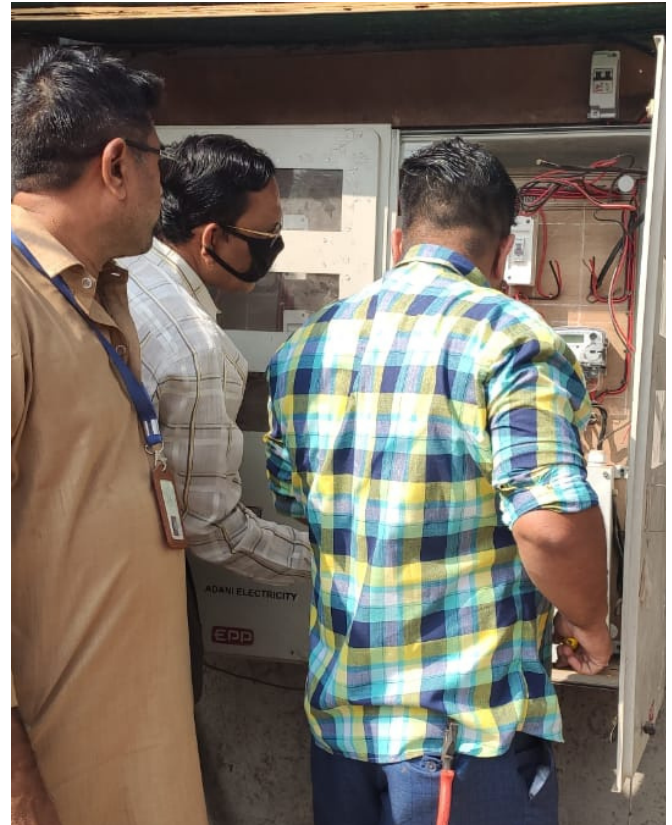
Officials in process of fixing the metered electricity connection.
