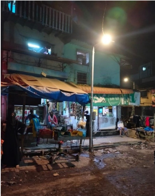
The streetlights installed at Rafi Nagar.
